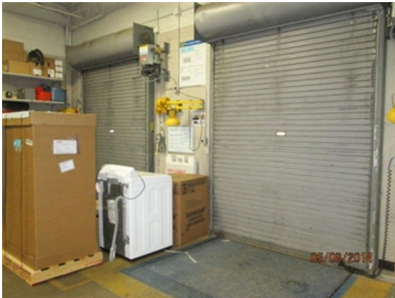
Freight Doors: Dock area freight overhead door.
