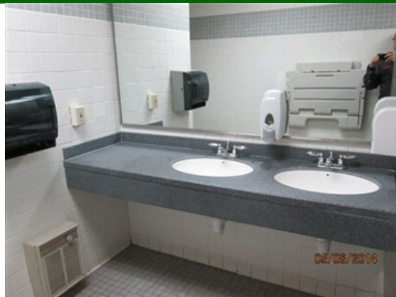
Bathrooms: Women's restroom vanity.
