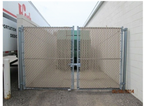
Fences / Enclosures: Fenced area for recycling compactor.
