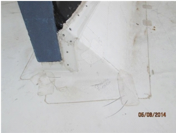
Roofing: Membrane flashing at parapet wall.
