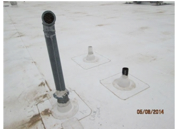
Draft Control/Vent: Typical roof penetrations.
