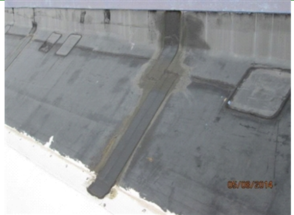
Attic Insulation: Backside of main parapet wall at north side.
