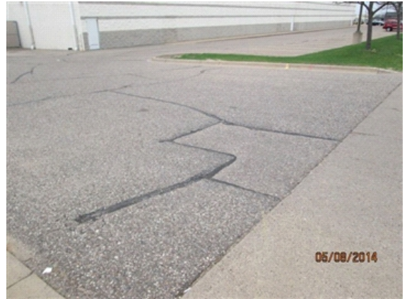
Parking Lot: Entrance to driveway area at the southeast corner.
