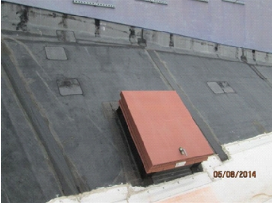
Parapet Wall: Hatchway into larger and higher parapet section.
