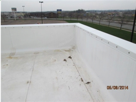
Attic Insulation: General view of roof at corner.
