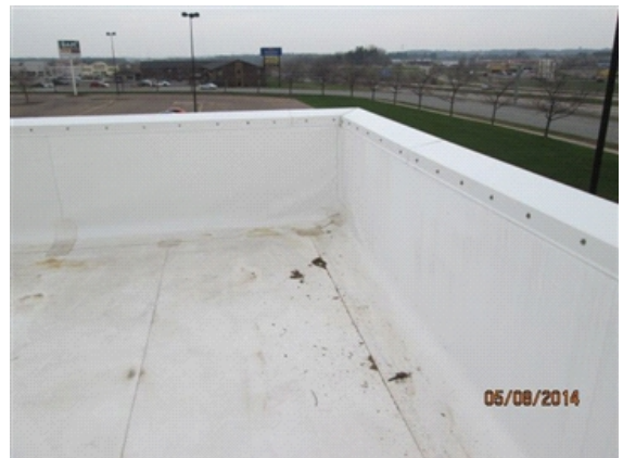
Parapet Wall: Parapet walls in northeast corner of roof.
