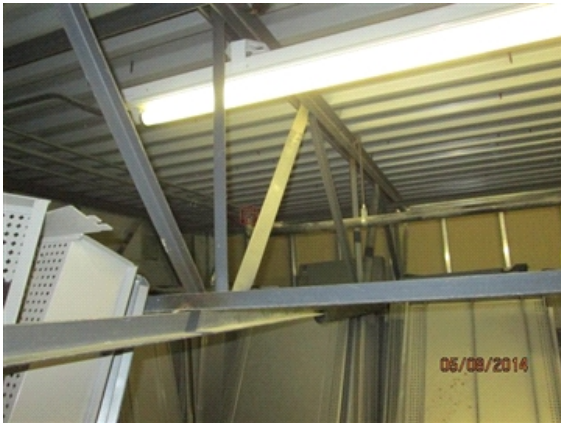
Structural Frame and Building Envelope: Detail of joist and decking.
