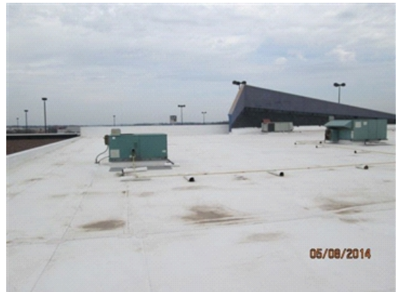
Attic Insulation: General view of roof looking north.
