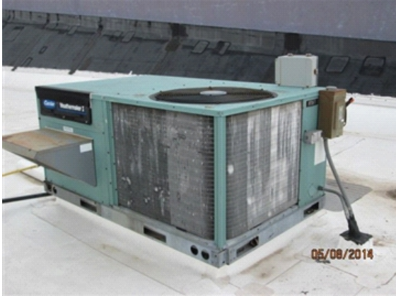
Heating (Trane units): Trane RTU unit.
