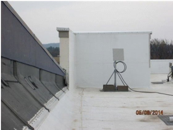
Roofing: View across the north face looking east.
