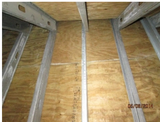
Attic Framing/Sheathing: Framing of front parapet wall - metal studs and plywood.
