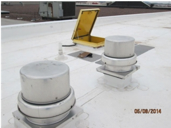
Attic Insulation: General view of roof looking south.
