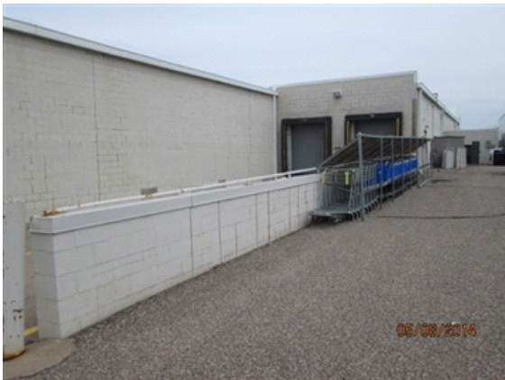
Retaining Walls/Landscaping: Dock area retaining wall.
