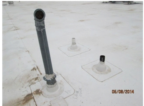
Flashing/Valleys: Typical roof penetrations.
