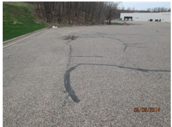
Grading / Drainage: South side of property slopes to the west to a drainage area and catch basins.
