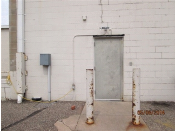
Main Doors: Main service door at shipping and receiving area.
