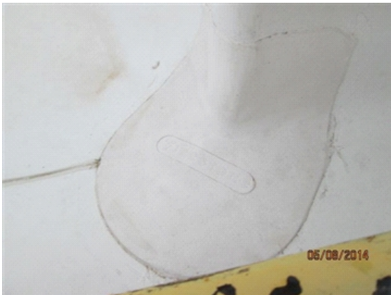
Flashing/Valleys: Membrane roof joint. Typical, in good condition.
