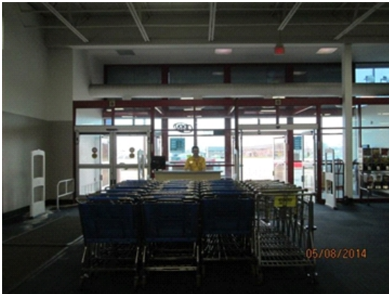
Fenestration Systems: View of windows from the inside of the building.
