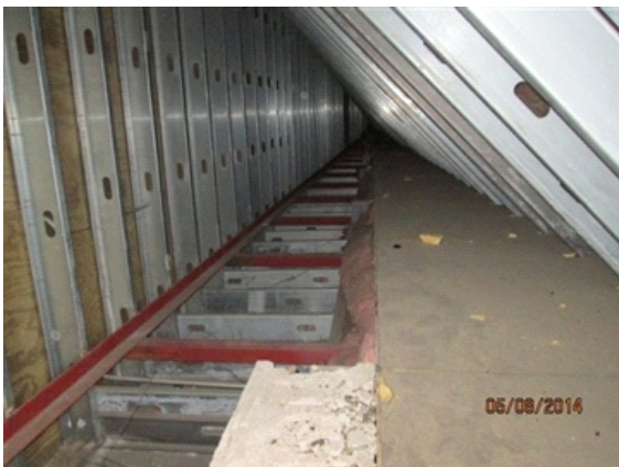
Attic Framing/Sheathing: Framing of front parapet wall - metal studs and plywood.
